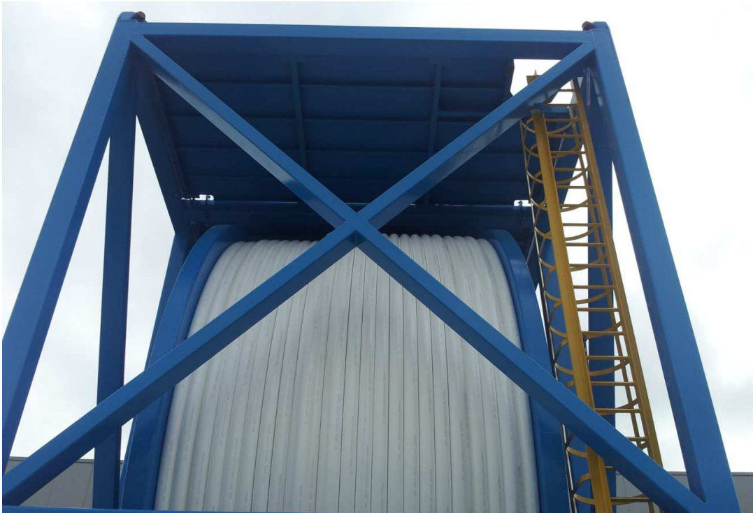
Figure 4: Ladder and covered roof.
